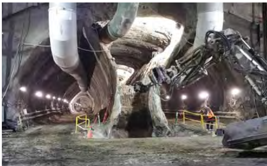
SEM cavern center-drift excavation.
