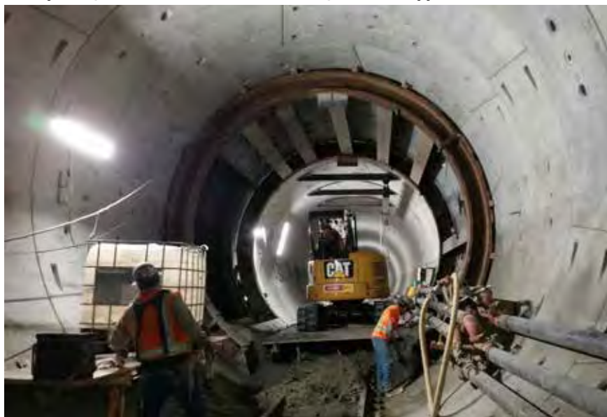
Crosspassage excavation with hamster cage tunnel support.
