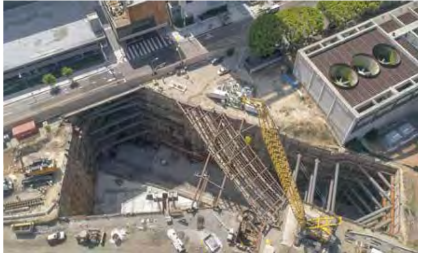
2nd and Hope Station excavation.
