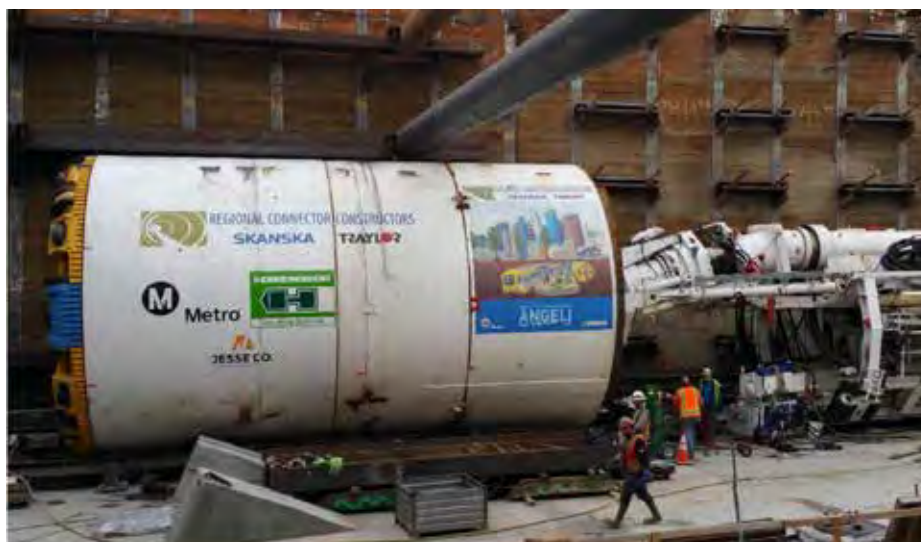
TBM Angeli at launching shaft.
