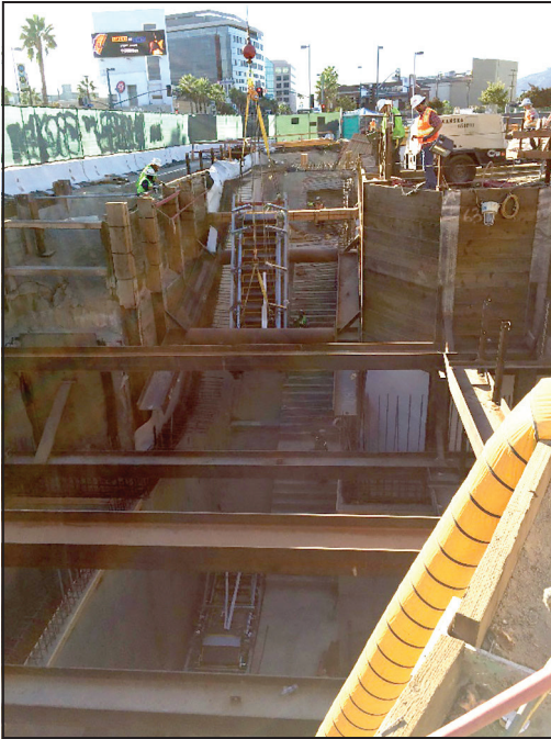
Figure 7. Installing escalators
