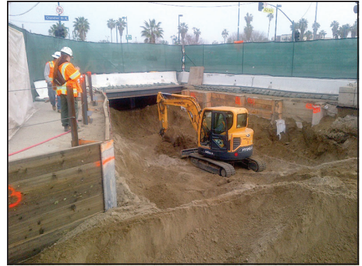
Figure 5. Small size excavator for low headroom excavation
