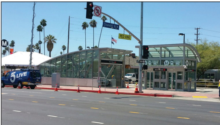
Figure 8. North Hollywood Station west entrance completed
