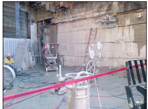
Figure 6. Cutting 4-foot thick reinforced concrete KOP
