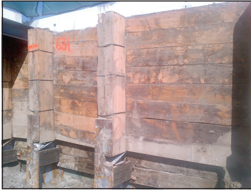
Figure 4. Extended existing soldier piles for reutilization
