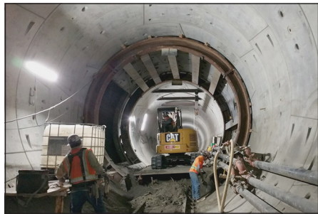
Figure 9. Crosspassage excavation with hamster cage tunnel support
