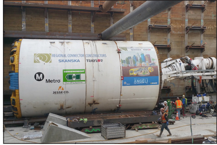
Figure 7. TBM Angeli at launching shaft
