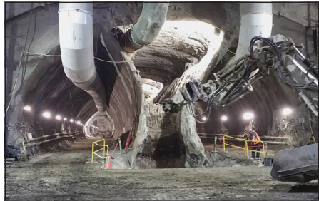
Figure 10. SEM cavern center drift excavation
