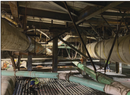
Figure 10. Construction of C&C tunnel roof
