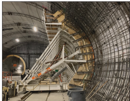
Figure 7. SEM cavern prefabricated wall form
