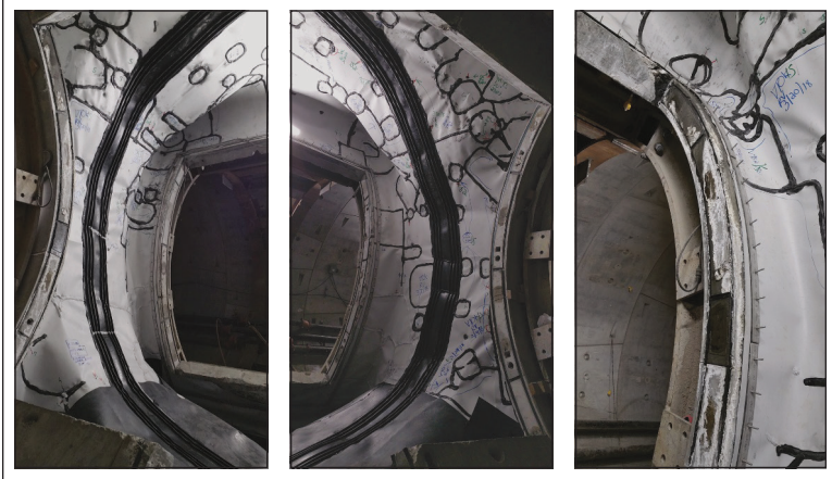
Figure 5. Crosspassage HDPE waterproofing system
