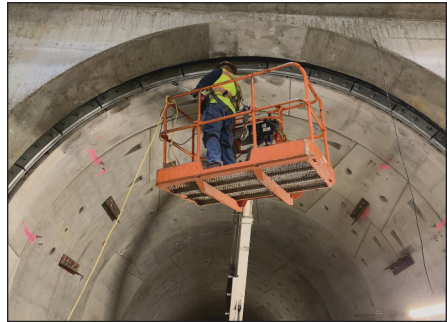
Figure 4. Omega seal installation
