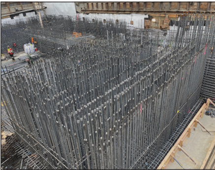
Figure 14. Threaded rods for future overbuild
