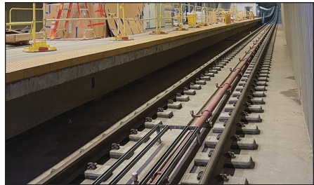
Figure 22. Under-car deluge systems
