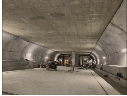
Figure 9. Completed SEM cavern at track level
