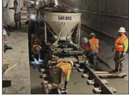
Figure 20. Infill concrete placement
