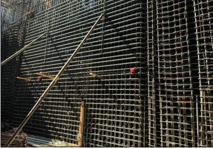
Figure 12. Example of station wall rebar
