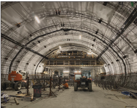
Figure 6. SEM cavern HDPE installation
