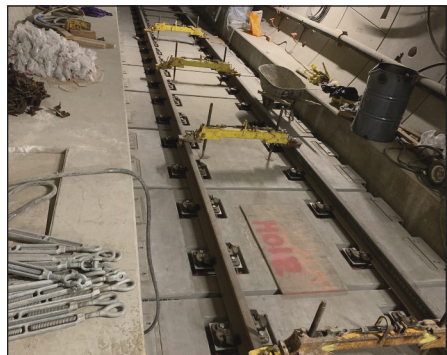
Figure 18. Completed floating slab track
