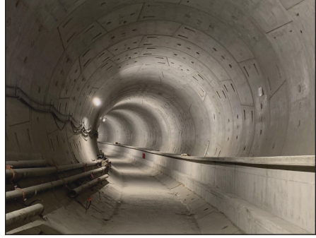
Figure 2. Completed emergency walkway
