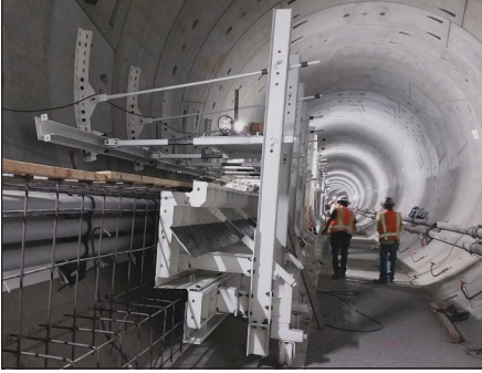
Figure 1. Emergency walkway prefabricated forms
